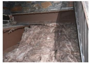
Disintegrated insulation has been replaced with materials that allow the building to breath as well as insulate.
